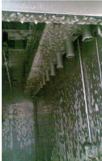
cleaning air duct
